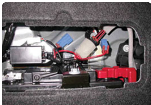
Primary battery in trunk with blue transit isolation connector
